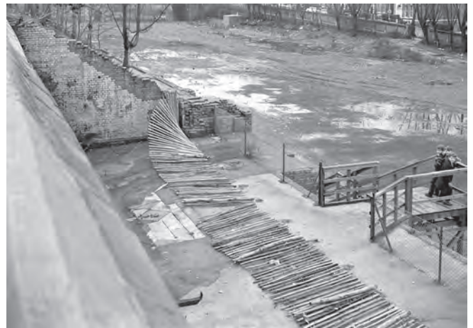
The subway terrace on the Southwark side - note some original diamond paving is visible. Photo reproduced by permission of Tony Harden from his collection
